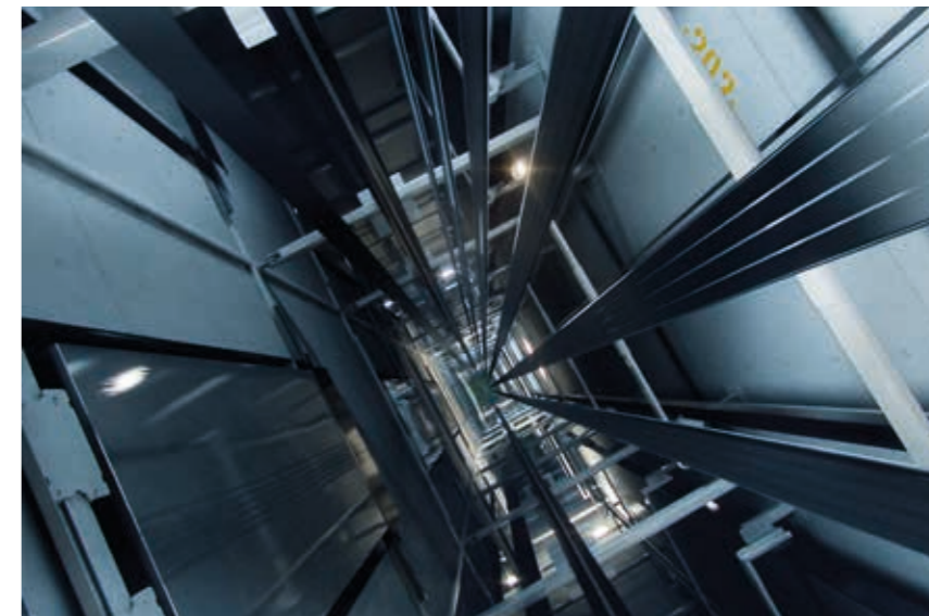
KONE UltraRope can enable future elevator travel heights up to 1,000 meters – twice as high as what is possible with today's technology.
